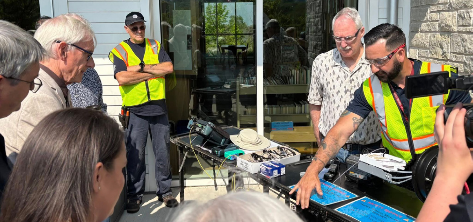
Gov. Tony Evers views a fiber optic splicing demonstration in Egg Harbor as part of a visit spotlighting the Broadband Infrastructure Program. Grants were awarded to areas of the state lacking access to 100/20 wireline connections.
